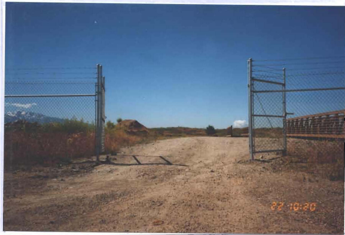
19. Photo looks south from 500 South street at the northern access to the RRD and its gate. A camera monitors access through this gate. Photo 31 of 31.
